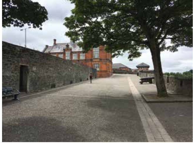
Masonic city wall: door in wall we used is on the left
