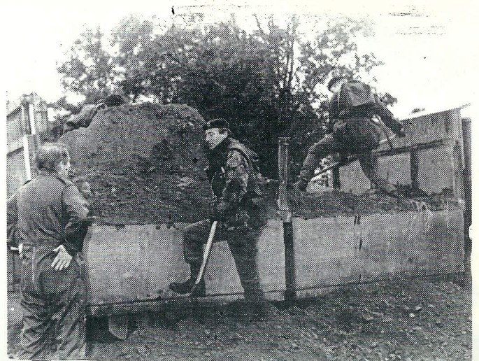
Of course, being a TA Officer, I'm quite used to this.
