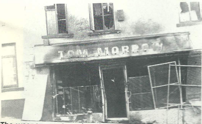
The weapon most used against business premises is the 'Blast Incendiary Device'—normally explosives and an inflammable liquid combined—the results can be devastating.
